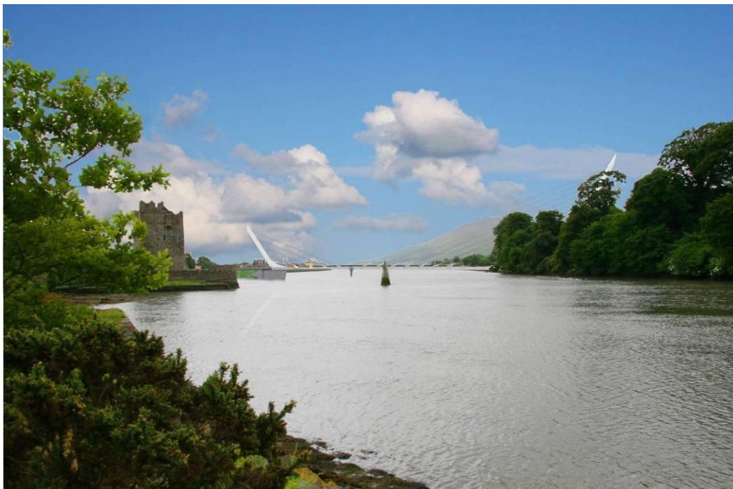
Plate 3.4 View from A2 on Newry side of Narrow Water Castle (Closed Position)
