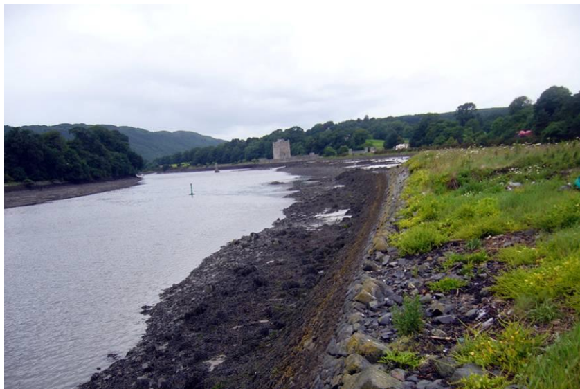
Plate 10.19 Training wall partially enclosing 'The Gut' on the County Down side.
