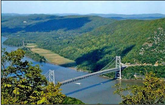
Bear Mountain Bridge in New York State.
